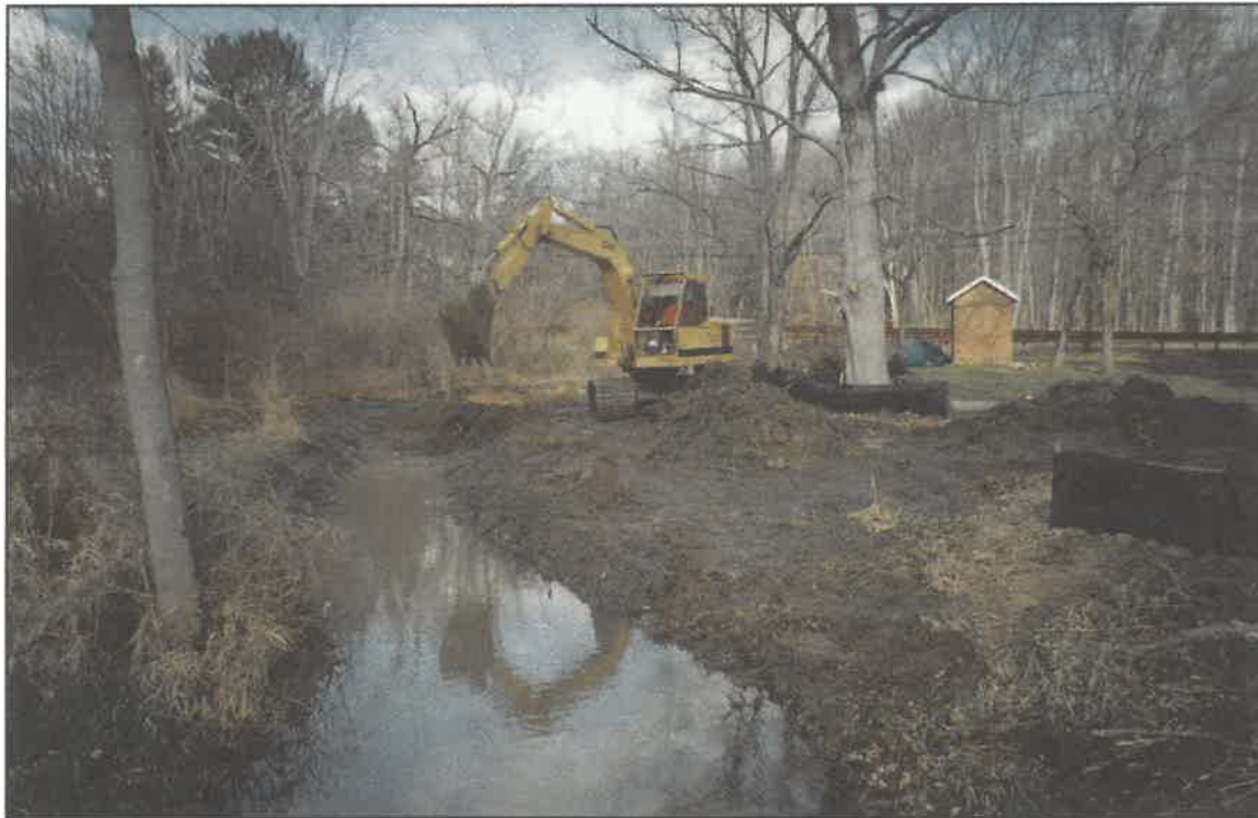
The stream restoration project is under way.
