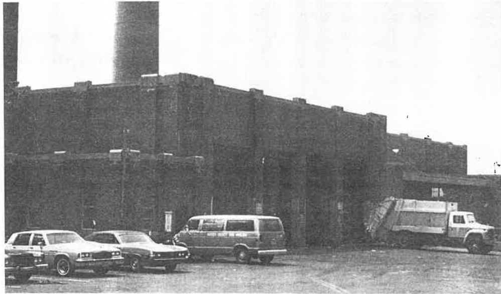
Trucks dispose of municipal solid waste at the Greenwich transfer facility for transfer to 65 yd 3 vehicles for disposal at Milford landfill, 45 miles away.
